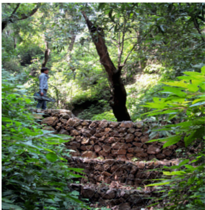
Loose boulders check dam
